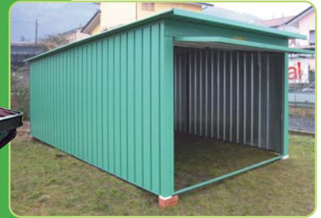
Garage in ferro e lamiera
